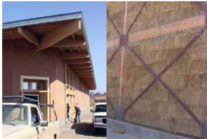
Figure 2. View of Entry and Detail of Straw Bale Wall
