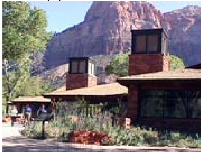
Figure 3. View of "Cool Towers" and Entry Courtyard
