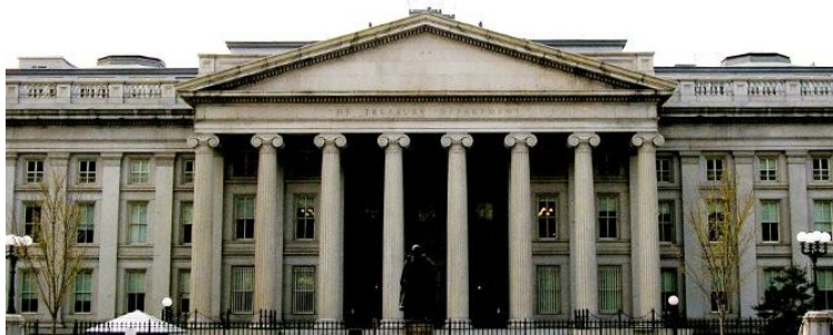
The iconic U.S. Treasury Building earns LEED Gold certification
