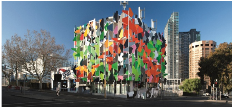
Global green building: Studio 505's Pixel building in Australia is LEED Platinum (Photo credit: John Gollings)
