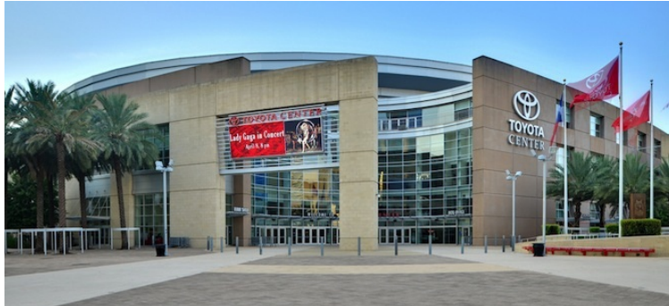
The LEED Silver Toyota Center in Houston, home of the Rockets. Credit: euthman via Flickr
