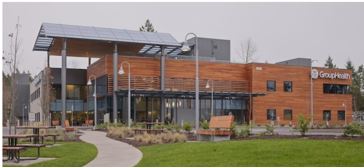
The Group Health Puyallup Medical Center in Puyallup, Wash., LEED Gold. Credit: Sozinho Imagery
