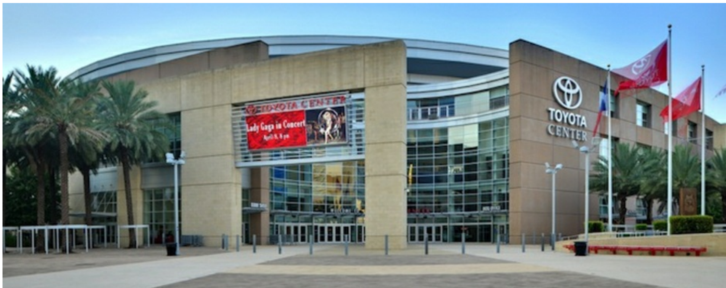
The LEED Silver Toyota Center in Houston, home of the Rockets. Credit: euthman via Flickr
