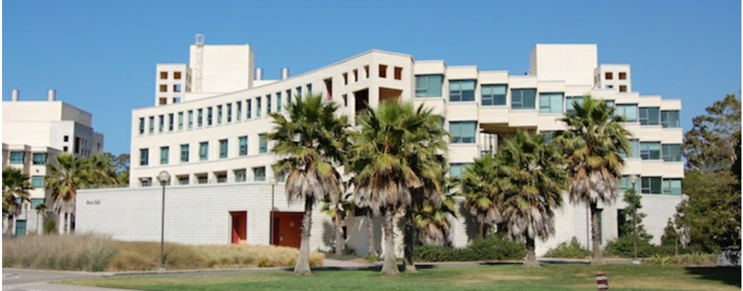
Bren Hall at the University of California, Santa Barbara has earned double LEED Platinum certification.
