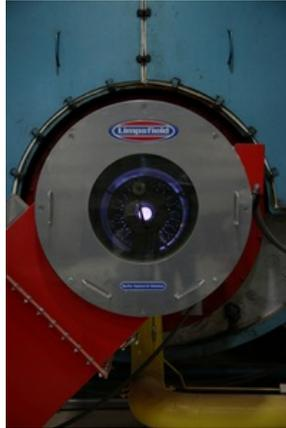
**This boiler is low NOx. In partnership with Arizona State University, Intel has installed an experimental algae biofuel demonstration unit to capture boiler emissions of carbon dioxide and create biofuel.**
