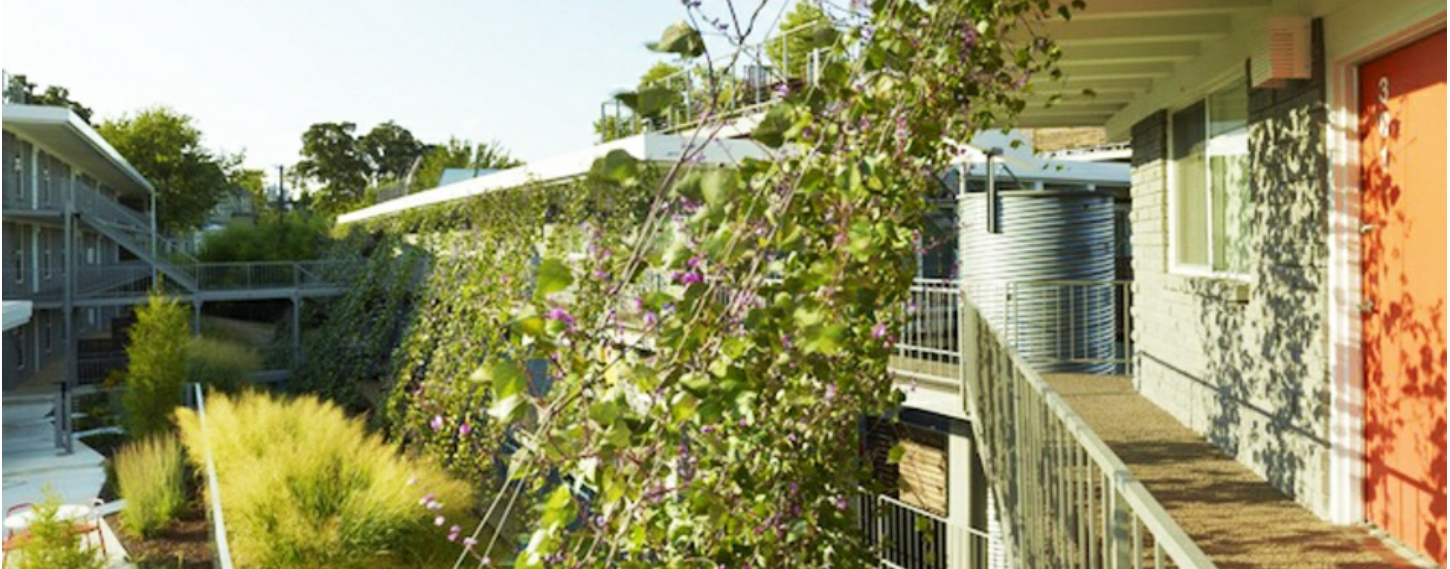
Eco Modern Flats, a multi-family project, in Fayetteville, AR - Photo by Timothy Hursley
